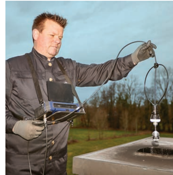
The carrying strap system leaves both hands free for safe inspection from the roof.
